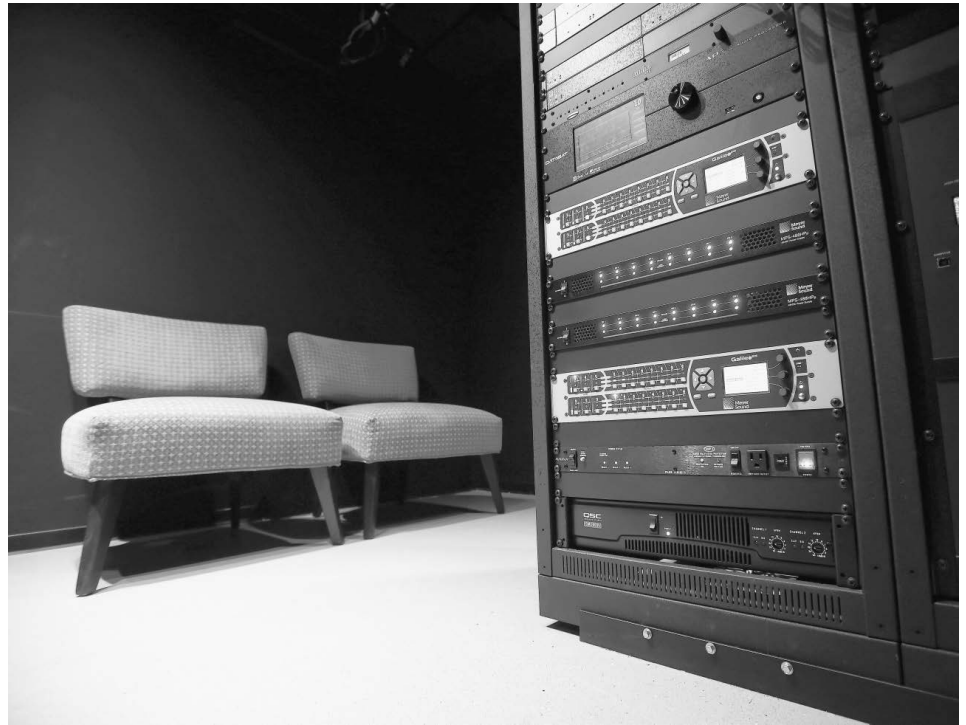
THE CONTROL PANEL inside the projection room at United Talent Agency’s private screening room.
